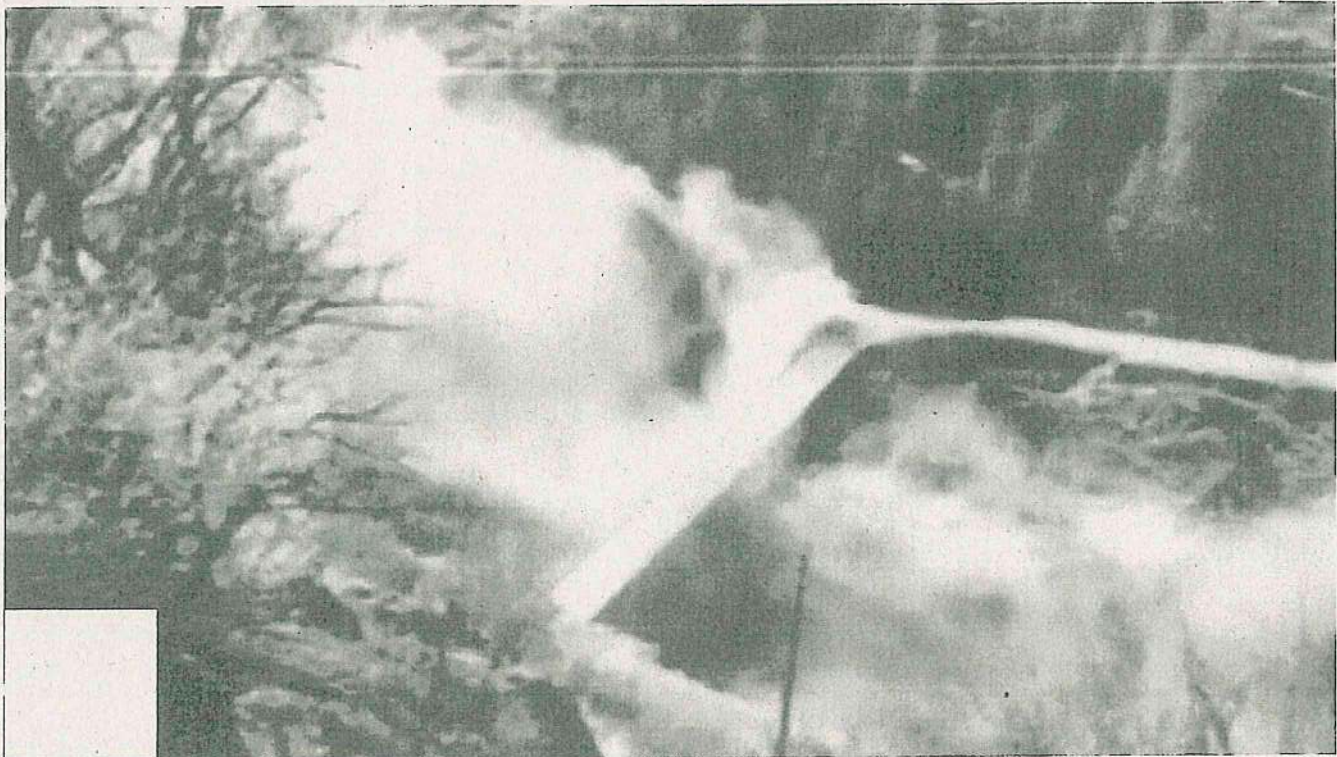
The moment the deluge of water washed away parts of the dam
